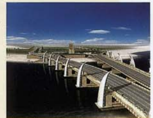
The Gateway Bridge - building the road to The Palm, Jumeirah
